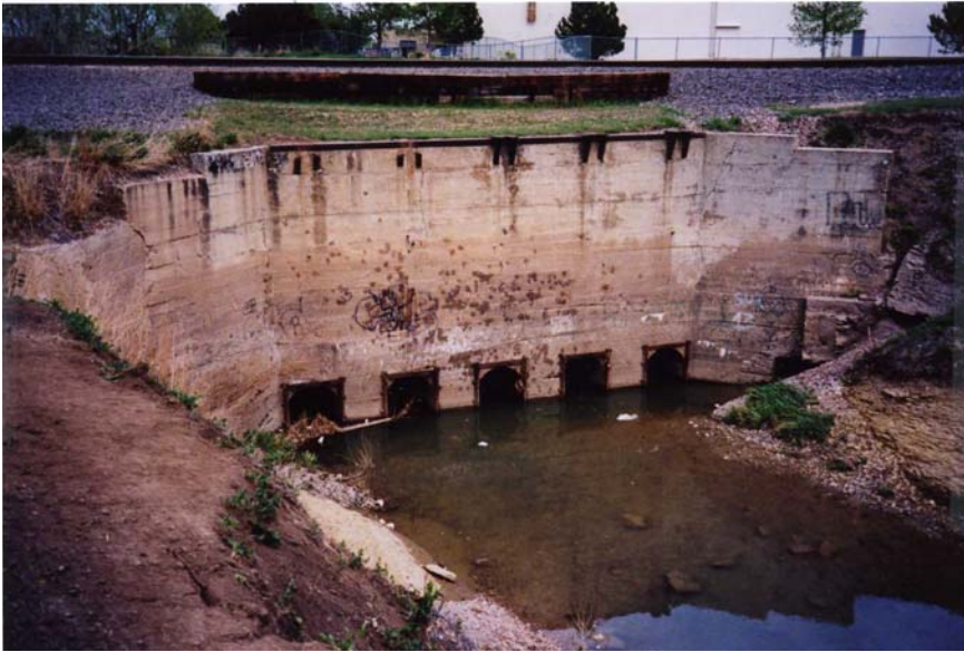
North I-25 North Loveland Ditch 5-9-06 Pg. 55
