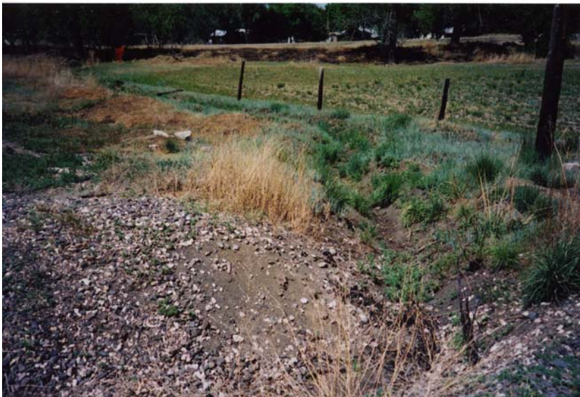
North I-25 C8 Ditch E of Site 20—N
