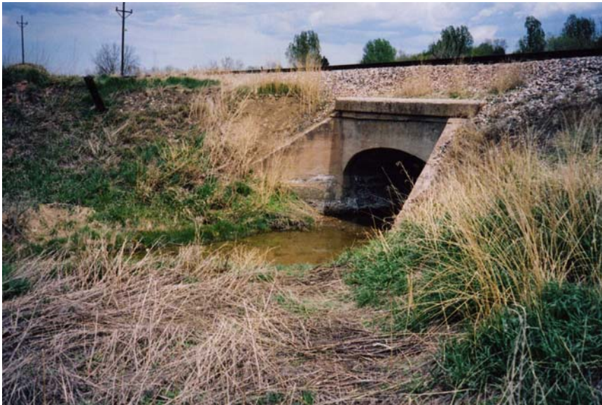
North I-25 A24 5-9-06 Site 12—NE West side
