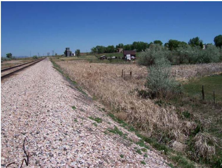
North I-25 Wetland 6A (east)—NE 5-24-06 Photo 7 Pg. 59
