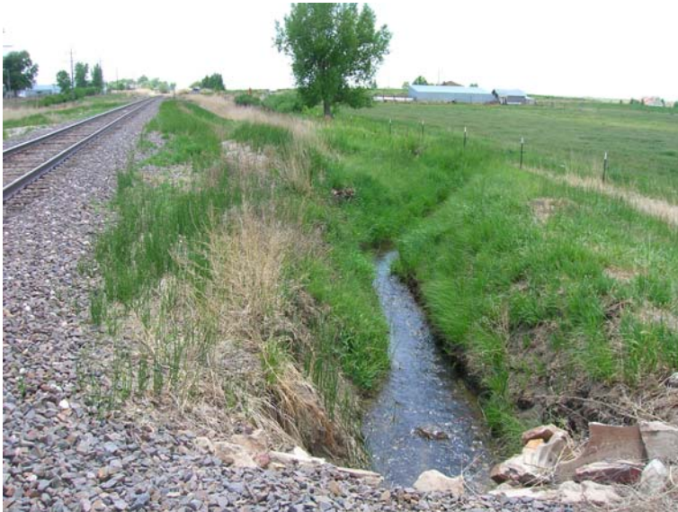
North I-25 1A (further south on tracks) 5-23-06 Drainage Ditch—SW
